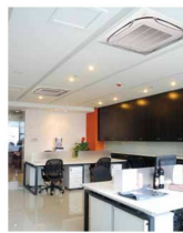
Ceiling Mounted Cassette (Round Flow with Sensing) Type
