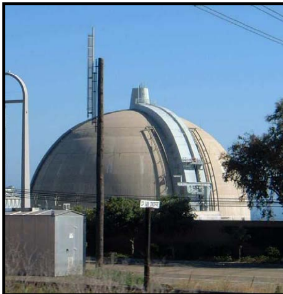
FIGURE 5-3. CONTAINMENT BUILDING AT SAN ONOFRE NUCLEAR GENERATING STATION, CALIFORNIA [FANCHI, 2002]
