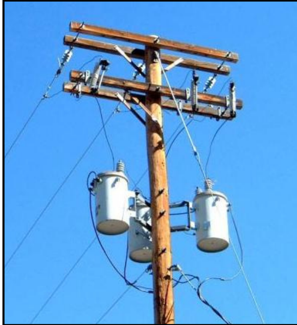
Figure 11-9. Pole-Mounted Transformer (Fanchi, 2003)
