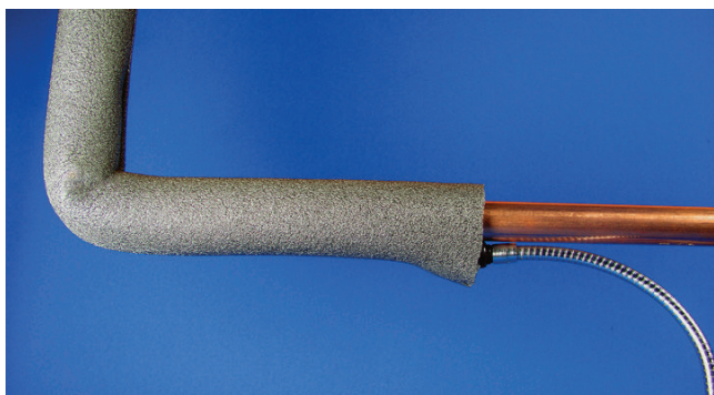
Figure 8.9 The probe of an electronic leak detector tucked underneath refrigerant pipe insulation sniffing for refrigerant leaks.
