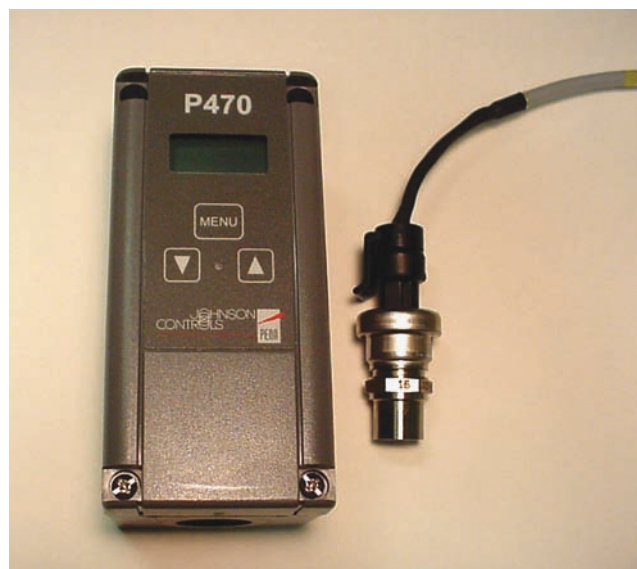
Figure 14.44 An electronic pressure control with a connecting pressure transducer. Courtesy Ferris State University. Photo by John Tomczyk
