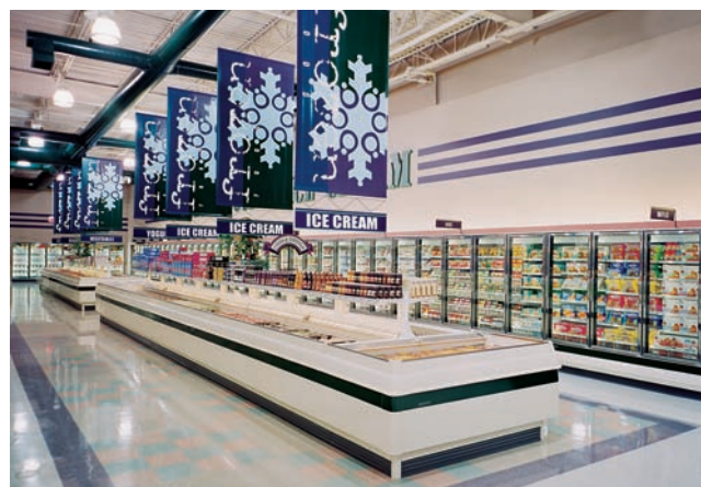
Figure 26.1(A) Display cases are used to safely store food displayed for sale. Some display cases are open to allow the customer to reach in without opening a door; some have doors. Closed cases are the most energy efficient. Courtesy Hill Phoenix
