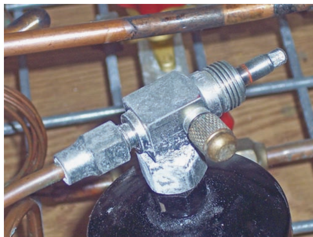
Figure 10.5 Liquid-line service valve located on the refrigerant receiver. Photo by Eugene Silberstein
