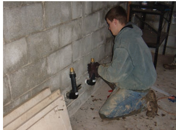
Figure 44.12(G) A technician working on the supply and return headers for the slinky ground loops that have entered the basement of the house. Courtesy Patrick Pung, Ferris State University HVACR Graduate
