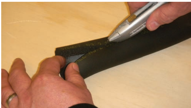
Figure 7.6 Pipe insulation being slit with a sharp razor knife.
