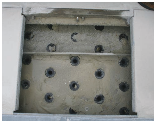
Figure 22.22 (A) Calibrated holes at the top of an induced-draft tower. The holes distribute the water over the fill material below. (B) Calibrated holes at the top of a cooling tower showing significant mineral deposits blocking water flow to the fill material. (B) Courtesy Ferris State University. Photo by John Tomczyk
