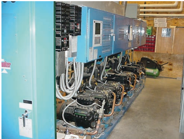
Figure 26.13 A parallel compressor system with load-matching capabilities. The microprocessor-based electronic controller is shown as part of the package. Courtesy Meijer Corporation, Big Rapids, MI. Photo by John Tomczyk
