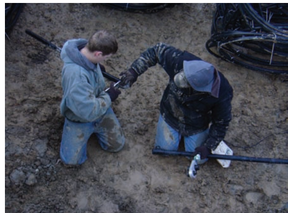
Figure 44.12(H) Two technicians applying custom vise-grip pliers around the plastic pipe to hold it firmly in place while getting it ready for the deburring process. Courtesy Patrick Pung, Ferris State University HVACR Graduate
