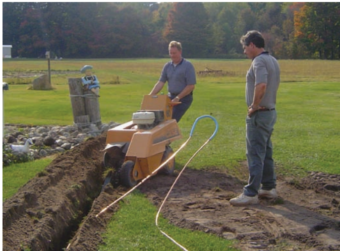
Figure 44.35 A trencher digging the trench for the refrigerant loop. Courtesy CoEnergies LLC, Traverse City, Michigan
