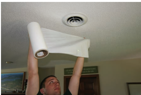
Figure 39.48(A) Tape off all supply registers with a duct sealing material such as Duct Mast or a high-quality painter’s masking tape and masking paper. Courtesy Ferris State University. Photo by John Tomczyk
