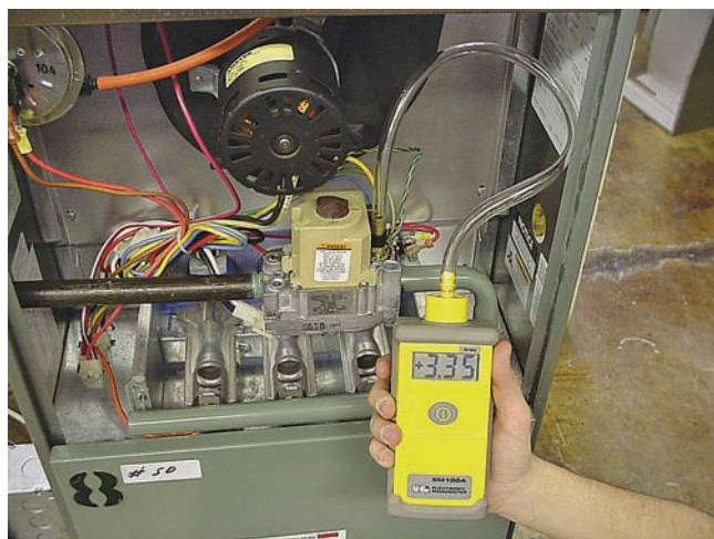
Figure 31.12 A digital manometer being used to measure gas pressure in inches of water column. Courtesy Ferris State University. Photo by John Tomczyk
