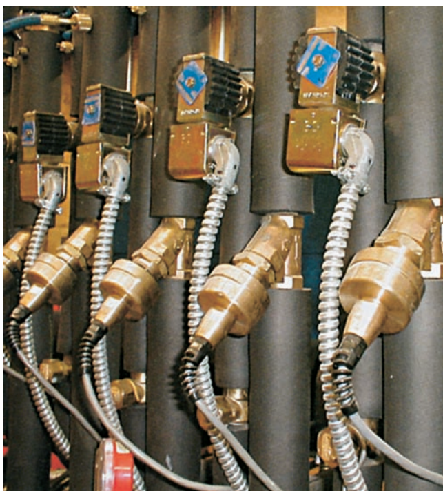
Figure 26.14(C) Modern step-motor-type, electronic evaporator pressure-regulator (EEPR) valves on the common suction line of a parallel compressor system. They react to a thermistor in the refrigerated case's evaporator discharge air. Courtesy RSES Journal
