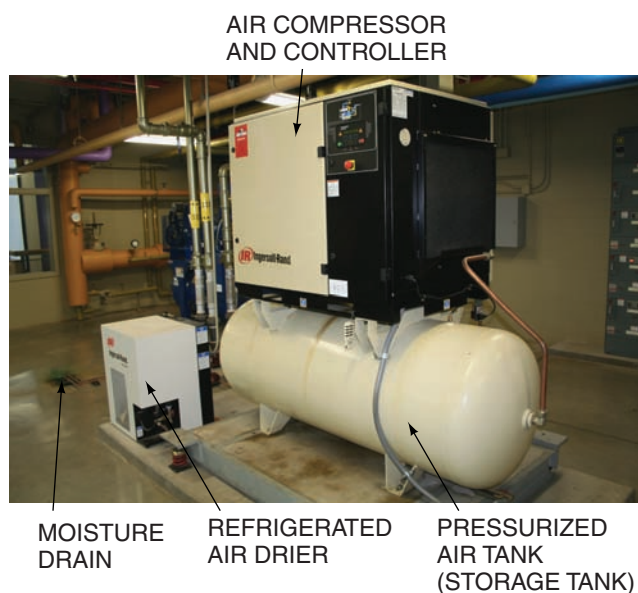
Figure 26.77 Refrigerated air drier with accompanying air compressor, controller, and pressurized air storage tank. Courtesy Ferris State University. Photo by John Tomczyk
