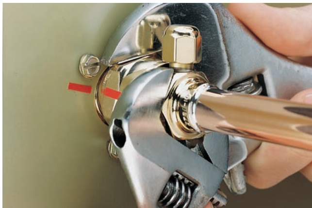
Figure 38.48 Using two wrenches to tighten fittings—one to hold the nut with the service tap on it and one to turn the movable nut next to the cabinet. Courtesy Aeroquip Corporation
