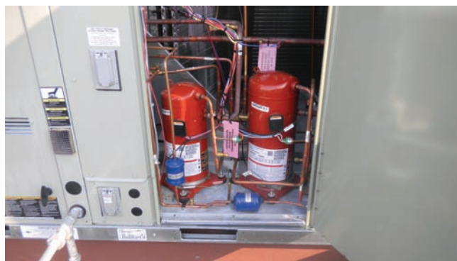
Figure 50.2 A 10-ton, two-circuit piping arrangement with two 5-ton compressors. Photo by Eugene Silberstein
