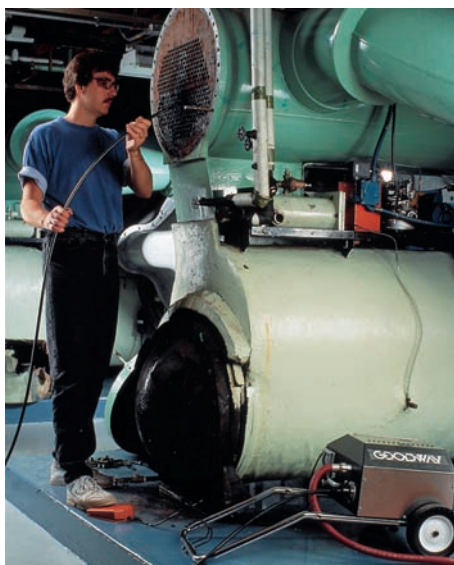
Figure 47.18 Cleaning the tubes in a condenser by using a power brush and flushing with water. Courtesy Goodway Tools Corporation
