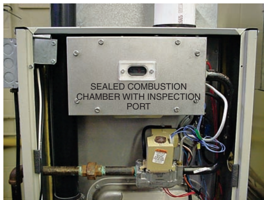
Figure 39.56(B) A sealed combustion chamber with a flame inspection port on a high-efficiency furnace.
