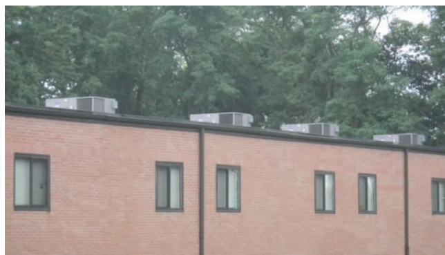
Figure 50.3 This building has several rooftop units to serve the various areas in the structure. Photo by Eugene Silberstein
