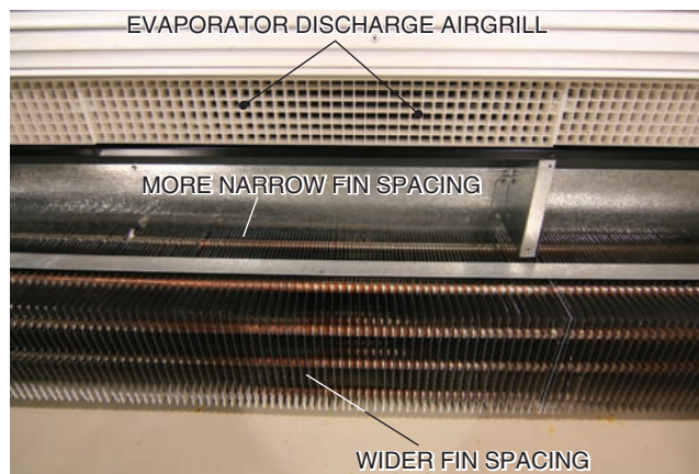
Figure 21.15 (A) A finned-tube evaporator for a medium-temperature commercial refrigeration case. (B) Finned-tube evaporator for a low-temperature, commercial, well-type freezer. Notice the two different fin spacings in the freezer's evaporator.
