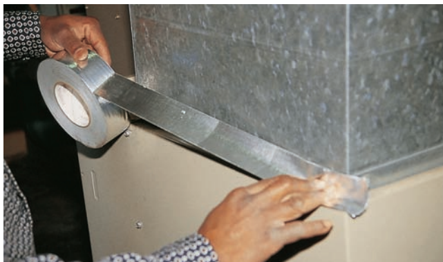
Figure 37.37 A taped duct connection. Photo by Bill Johnson
