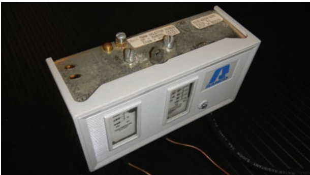
Figure 14.64 This high-pressure control is considered an electromechanical control. Photo by Eugene Silberstein
