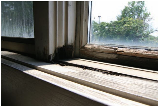
Figure 39.31(A) A window where condensate has run down the glass and rotted the bottom structure of the window because of thermal bridging. Courtesy Ferris State University. Photo by John Tomczyk
