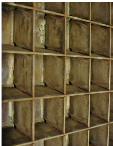
Figure 27.40 Weep holes between cells on the evaporator. Courtesy Ferris State University. Photo by John Tomczyk
