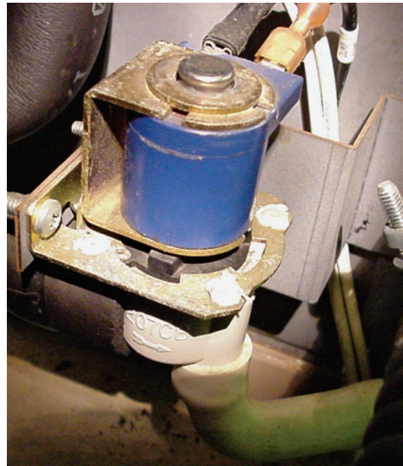
Figure 27.33 An electric, solenoid-operated water dump valve. Courtesy Ferris State University. Photo by John Tomczyk
