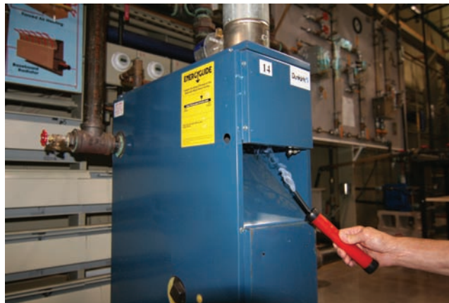
Figure 39.55(A) A technician using a chemical smoke generator in the vicinity of the draft diverter on a standard-efficiency furnace to look for smoke pulling into the diverter and drafting upward.
