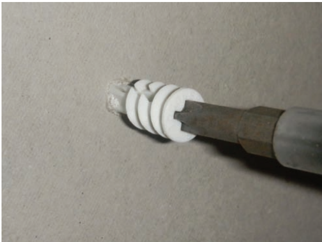
Figure 6.27 Installing the self-drilling drywall anchor. Photo by Eugene Silberstein
