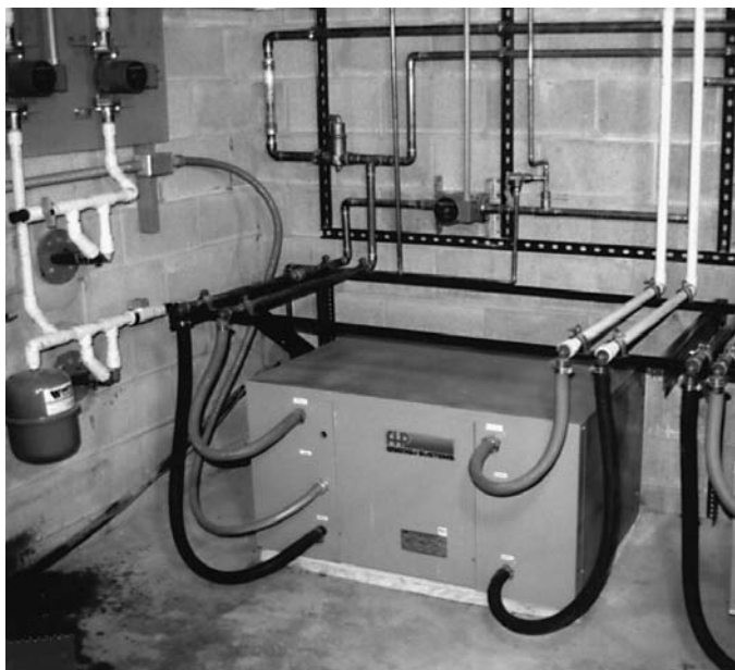
Figure 44.25 A water-to-water heat pump installed as part of a hydronic heating system.
