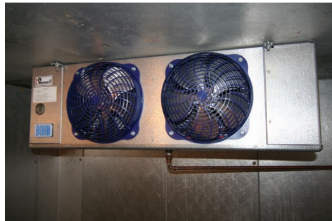
Figure 3.23 A typical refrigeration evaporator. Courtesy Ferris State University. Photo by John Tomczyk
