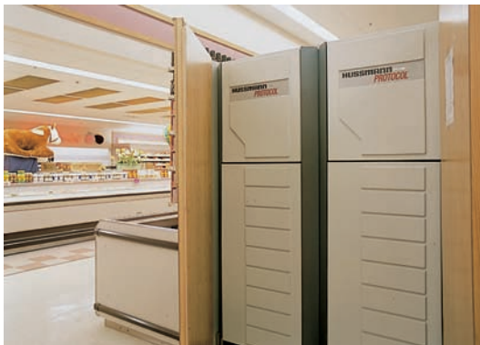
Figure 26.32 Unitary distributed refrigeration systems located close to the display cases they are refrigerating. Courtesy Husmann Corporation
