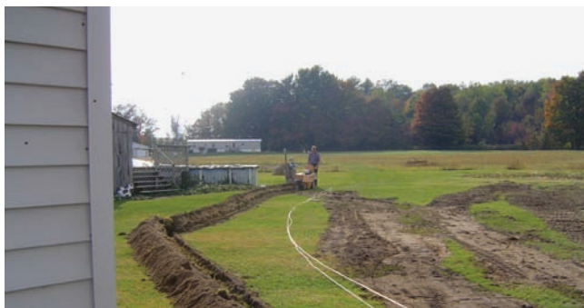
Figure 44.30 Polyethylene plastic-coated pipe being readied to be buried in a trench. Courtesy CoEnergies LLC, Traverse City, Michigan
