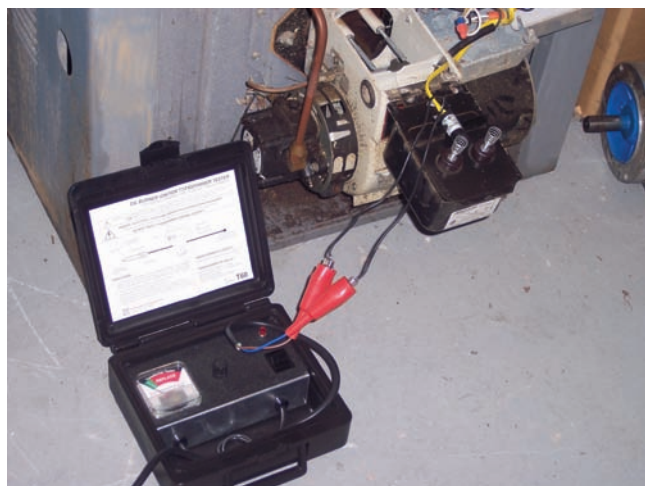
Figure 32.64 Ignition transformer tester connections. Courtesy Oilheat Associates, Inc. Photo by John Levey
