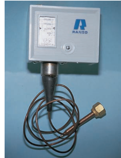
Figure 25.29 The low-ambient control used to open the contacts on a drop in head pressure to stop the condenser fan.
