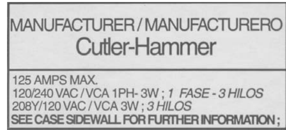
Figure 18.4 A nameplate on an electrical panel used for a power supply. Photo by Bill Johnson
