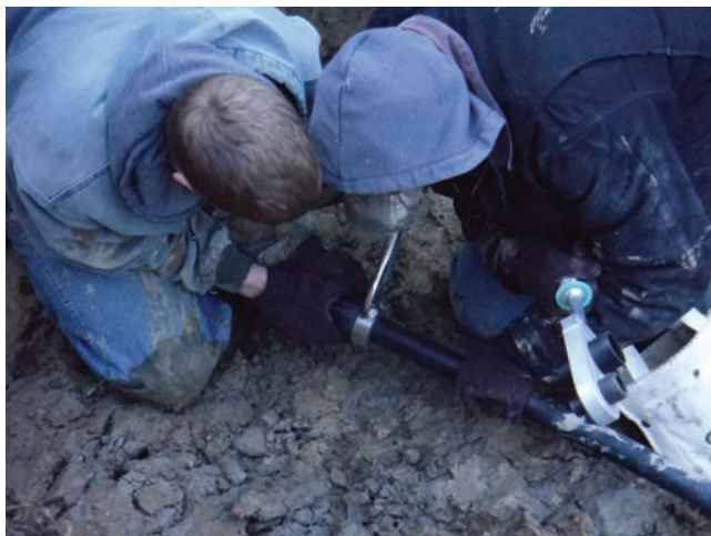
Figure 44.12(I) Plastic pipe being pushed into the coupling tee by two technicians. This process is performed after the heating of the plastic pipe and coupling tee is completed and the fusion iron is removed from the piping. Courtesy Patrick Pung, Ferris State University HVACR Graduate
