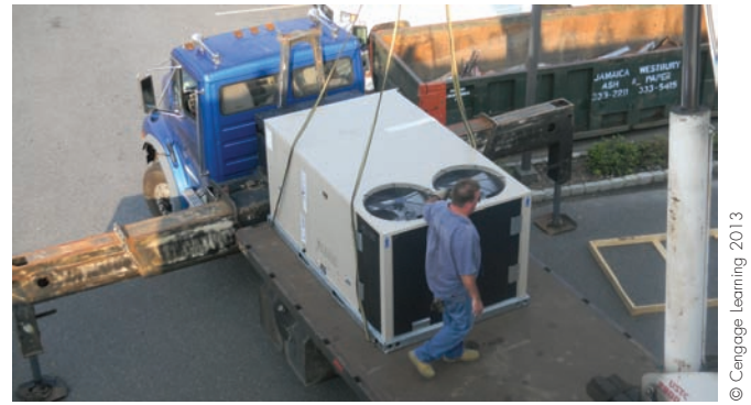
Figure 50.6 Rooftop unit with multiple condenser fans.
