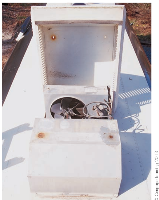
Figure 46.7 The case lifts off the roof-mount unit. Photo by Bill Johnson
