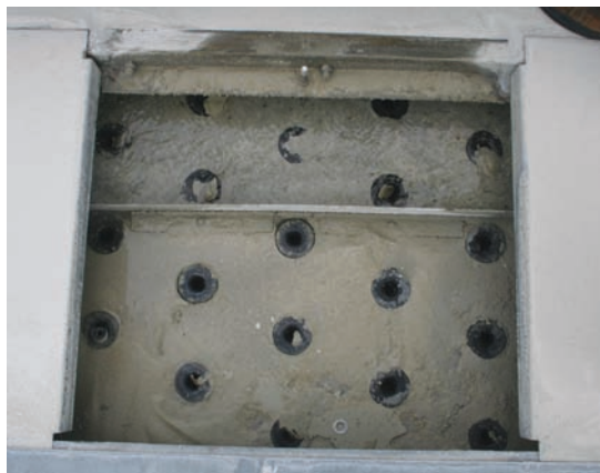
Figure 48.25 (A) Calibration holes for distributing water in the tower are enlarged due to rust. Most of the water is running down the right side of the tower. (B) Calibrated holes on top of a cooling tower showing significant mineral deposits blocking water flow to the fill material.
