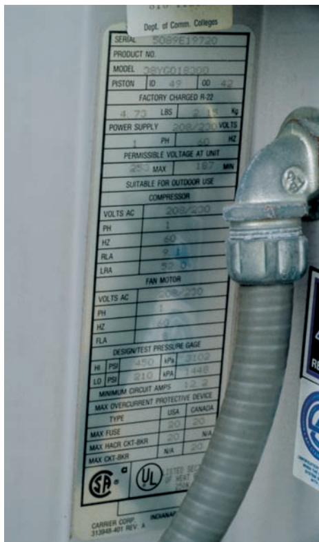
Figure 40.20 A condensing unit nameplate. Photo by Bill Johnson
