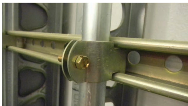
Figure 6.33 Steel channel and pipe clamp used to hold piping material. Photo by Eugene Silberstein
