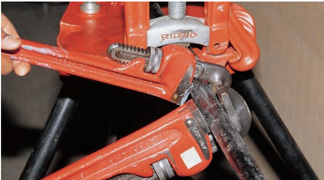
Figure 7.72 Holding the pipe and turning the fitting with pipe wrenches.
