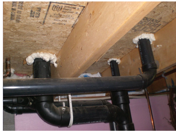
Figure 39.36(A) Insulating foam sealant sealing air leaks where plumbing fixtures penetrate through floors. Courtesy Fluke Corporation
