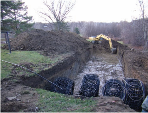
Figure 44.12(C) Four slinky ground loops in a freshly excavated trench waiting to be rolled out. Courtesy Patrick Pung, Ferris State University HVACR Graduate
