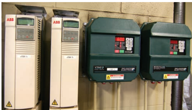
Figure 25.16(B) Four VFDs used to control the speed of a motor by varying the frequency delivered to the motor. Courtesy Ferris State University. Photo by John Tomczyk
