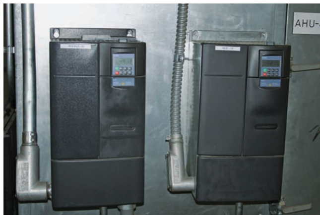
Figure 22.39 A variable-frequency drive (VFD) used in changing the voltage frequency to a motor. This will change the motor's speed in very small increments. Courtesy Ferris State University. Photo by John Tomczyk
