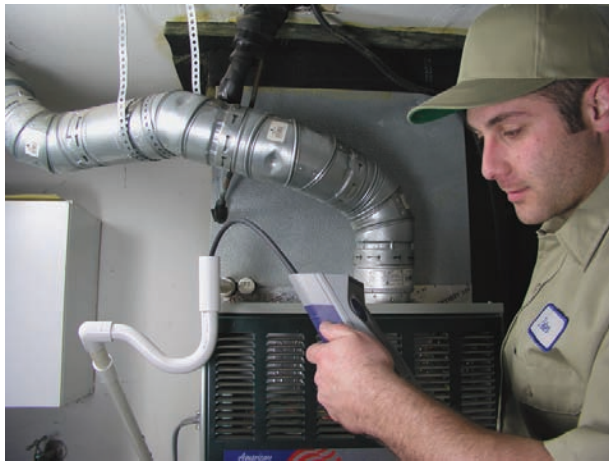
Figure 8.6 A service technician positioning an electronic leak detector at the drain opening of an evaporator drain.
