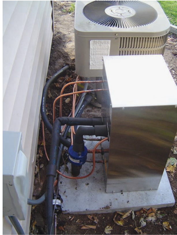
Figure 44.37 Insulated supply and return lines routed to the retrofitted air conditioner. Courtesy CoEnergies LLC, Traverse City, Michigan
