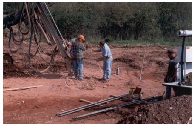
Figure 44.43 Diagonal drilling rig with workers feeding copper earth loop into small-bored hole. Courtesy Earthlinked Technologies, Inc.
