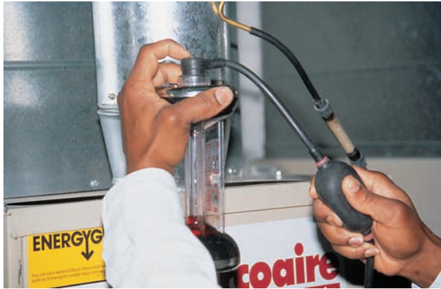
Figure 32.103 Performing a carbon dioxide test. Photo by Bill Johnson
