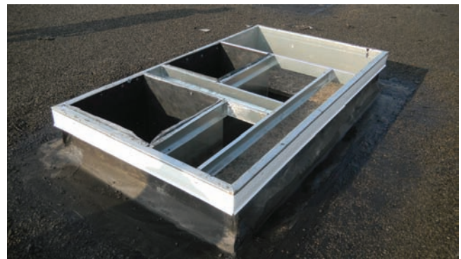
Figure 50.10 Typical roof curb. Photo by Eugene Silberstein
