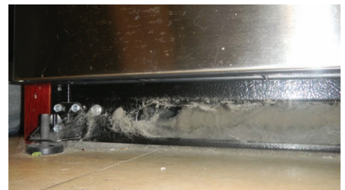
Figure 45.67 Induced-draft condenser located close to the floor collecting lint and dust. Photos by Eugene Silberstein
