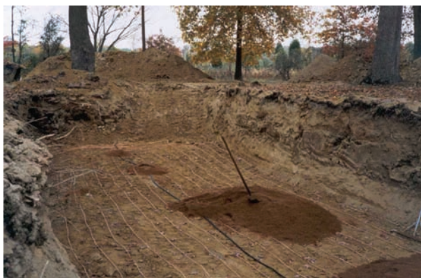
Figure 44.44 Horizontal earth loop installation. Courtesy Earthlinked Technologies, Inc.
