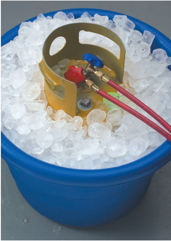
Figure 5.69 Ice bucket with refrigerant recovery tank being chilled. Courtesy Ritchie Engineering Company, Inc.
