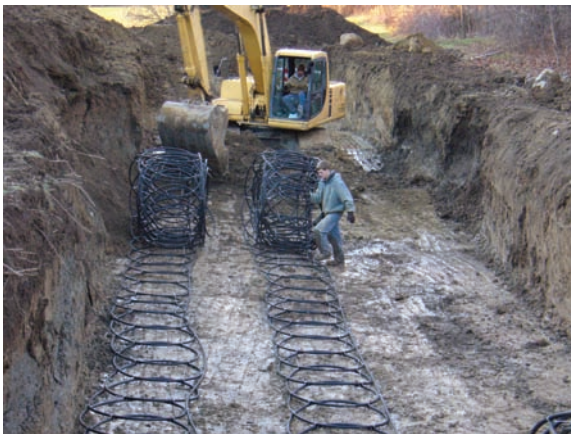
Figure 44.12(D) A technician in the process of rolling out a slinky ground loop. Courtesy Patrick Pung, Ferris State University HVACR Graduate
