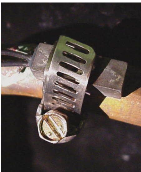
Figure 27.39 A thermistor on the discharge line of an ice maker. Courtesy Ferris State University. Photo by John Tomczyk
