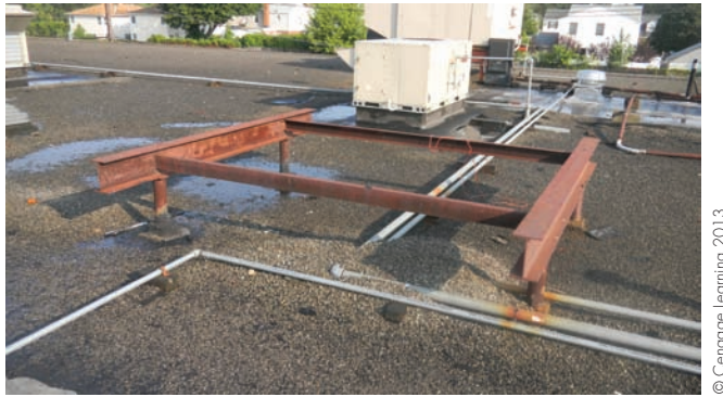
Figure 50.9 Steel rooftop support structure to keep unit above the snow level. Photo by Eugene Silberstein
