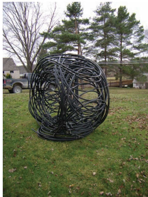
Figure 44.12(B) Prefabricated slinky ground loop waiting to be transported to the job site. Courtesy Patrick Pung, Ferris State University HVACR Graduate
