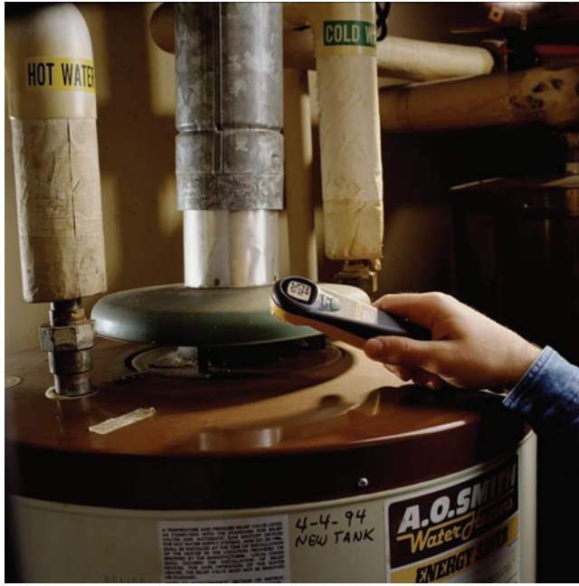
Figure 39.55(B) A technician checking a water heater with a digital carbon monoxide sensing meter. The meter will sense ppm CO coming into the home from backdrafting of the combustion appliance.
