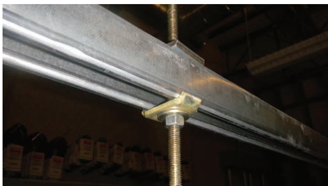
Figure 6.30 Threaded rod and steel channel used to make custom hangers. Photo by Eugene Silberstein
