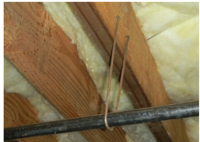
Figure 6.39 (A) A wire pipe hook. (B) Pipe hook installation. (B) Photo by Eugene Silberstein
