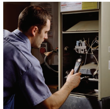
Figure 39.57 A technician checking a furnace for ppm carbon monoxide (CO) caused by spillage. Courtesy Fluke Corporation
