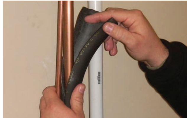
Figure 7.7 Pipe insulation being positioned over tubing section.
