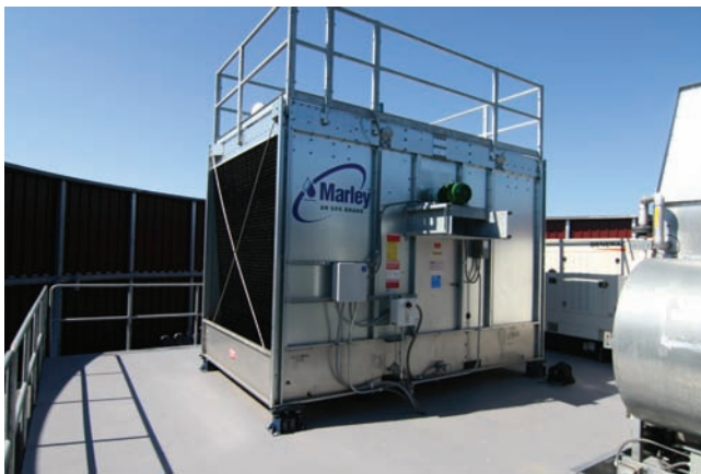
Figure 48.15(B) Modern cooling tower that was manufactured as a complete assembly and shipped to the job. Courtesy Ferris State University. Photo by John Tomczyk
