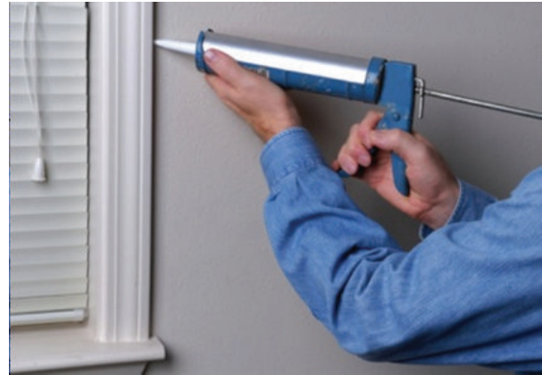
Figure 39.35(B) Caulking around windows to prevent air leakage. Courtesy Fluke Corporation
