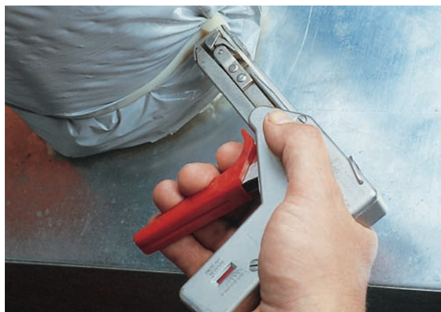
Figure 6.41 A system for fastening round flexible duct to a sheet metal collar. Courtesy Panduit Corporation
