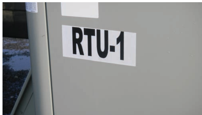
Figure 50.4 Typical identification label on a rooftop unit. Photo by Eugene Silberstein
