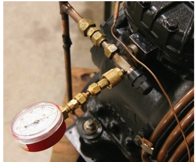
Figure 41.8 This short service connection is used on the high-side gauge port to keep too much refrigerant from condensing in the gauge line. Courtesy Ferris State University. Photo by John Tomczyk
