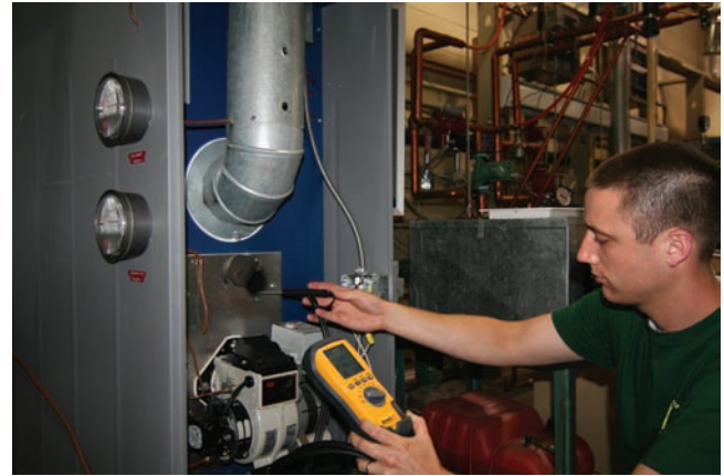
Figure 39.66 A technician taking an over-the-fire draft reading. Courtesy Ferris State University. Photo by John Tomczyk
