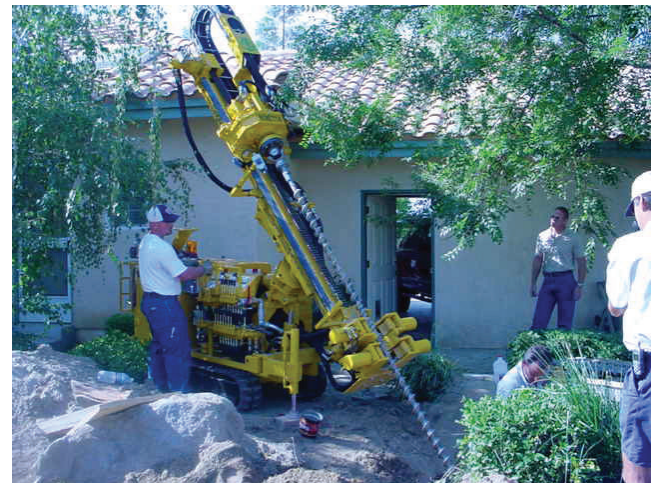
Figure 44.42 Diagonal drilling rig showing residence and small-bore drill. Courtesy Earthlinked Technologies, Inc.
