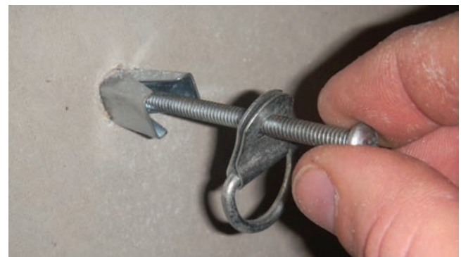
Figure 6.20 Inserting the folded toggle into the hole in the gypsum board. Photo by Eugene Silberstein
