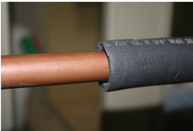
Figure 3.25 Suction lines should be well insulated to increase system efficiency and capacity and to prevent sweating. Courtesy Ferris State University. Photo by John Tomczyk
