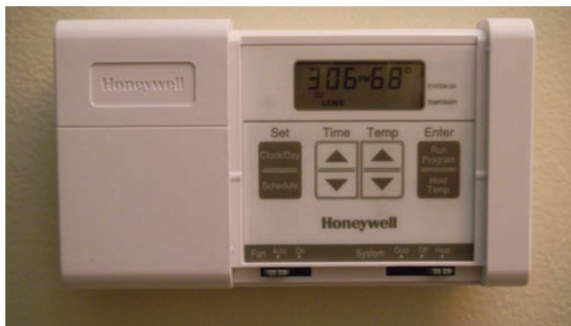
Figure 14.1 Both thermostats open on a rise in temperature, but they serve two different purposes. (A) The motor-winding thermostat measures the temperature of iron and copper while in close contact with the motor windings. (B) The space thermostat measures air temperature from random air currents. (B) Photo by Eugene Silberstein
