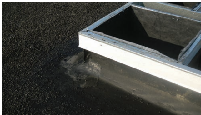
Figure 50.11 The curb must be properly sealed to prevent water leaks. Photo by Eugene Silberstein
