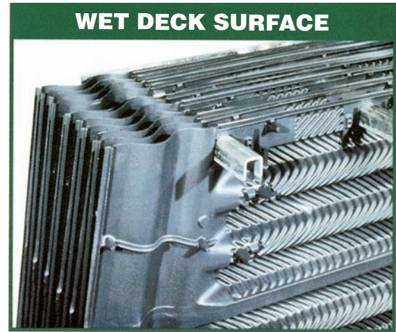
Figure 48.9 A PVC wet deck surface located below the prime surface coil in the closed-circuit cooling tower. Copyright, Baltimore Air Coil Company, 2003
