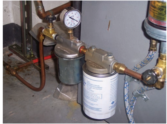
Figure 32.22 Dual in-line oil filtration. Courtesy Oilheat Associates, Inc. Photo by John Levey
