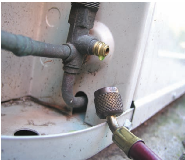
Figure 8.4 Oil on a service valve’s access port.
