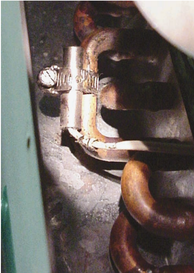
Figure 27.48 The condenser thermistor is an analog input to a microprocessor. Courtesy Ferris State University. Photo by John Tomczyk
