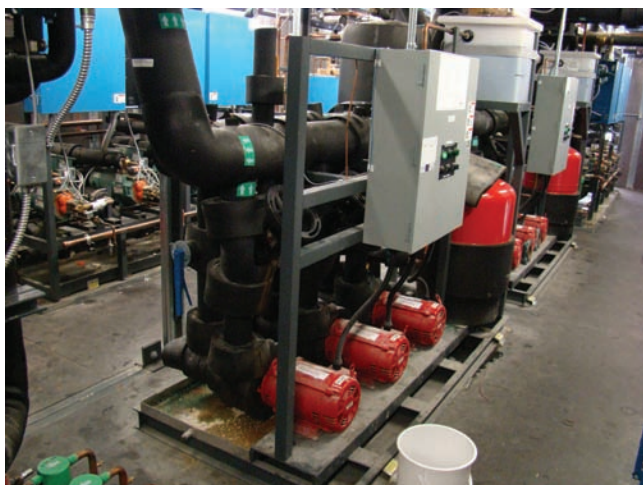
Figure 26.25(B) A secondary-fluid refrigeration system showing chillers and circulating pumps. Photo by Dick Wirz
