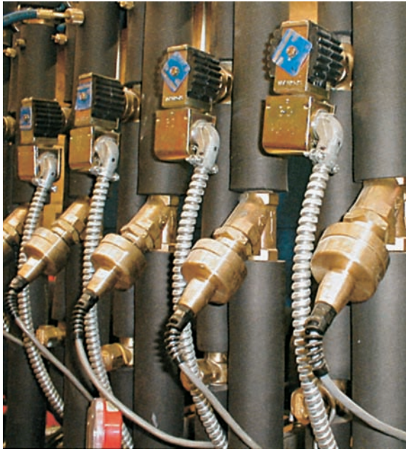
Figure 25.7 EEPR valves in suction lines on a parallel compressor system. Courtesy RSES Journal
