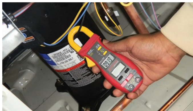
Figure 10.27 Taking a current reading at the compressor.
