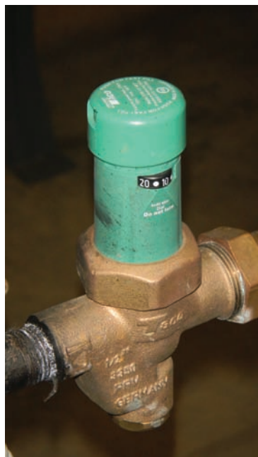
Figure 14.60 Adjustable water-regulating valve for a boiler. Photo by Eugene Silberstein
