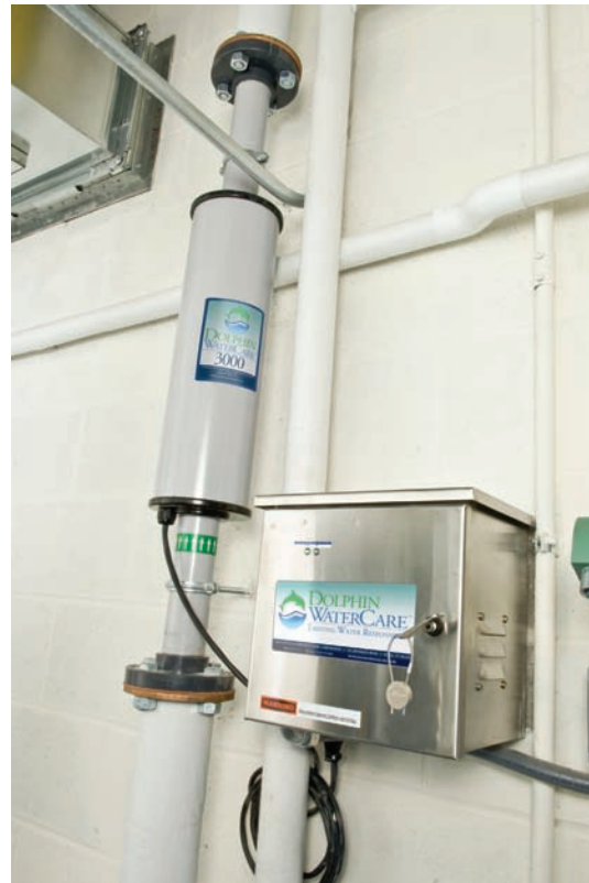
Figure 48.51(B) A signal generator and water treatment module installed in a working cooling tower.
