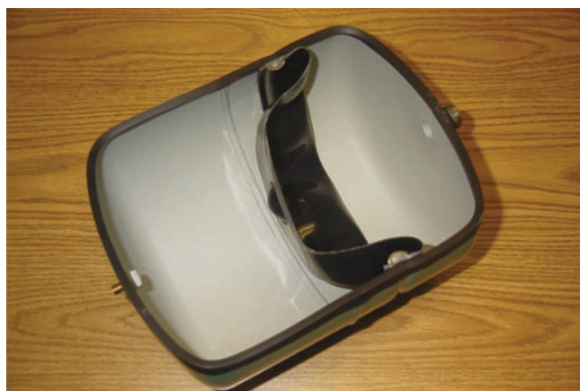
Figure 33.15 Cutaway view of a diaphragm-type expansion tank. Photo by Eugene Silberstein
