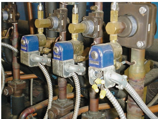
Figure 26.14(B) Evaporator pressure-regulating (EPR) valves on suction lines of a parallel compressor rack. As the EPR valves open and close according to the load on the cases, the pressure transducer on the common suction line will sense the change in pressure.
