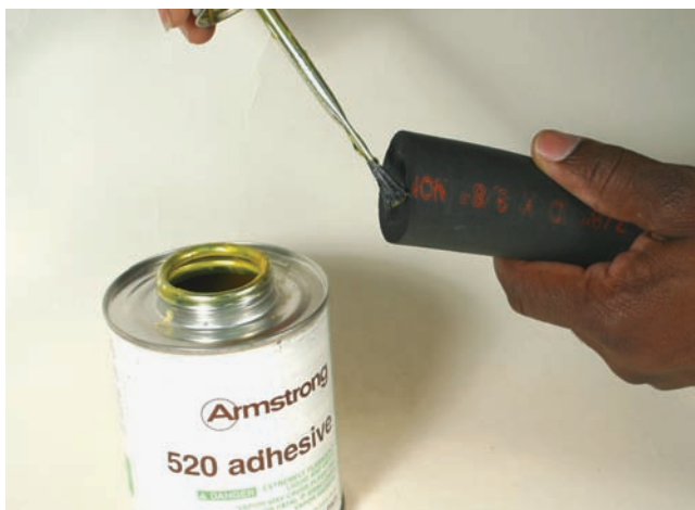
Figure 7.5 When joining two ends of tubing insulation, use an adhesive intended for this purpose.
