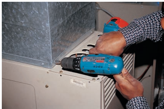
Figure 37.36 Fastening duct using a portable electric drill and sheet metal screws. Photo by Bill Johnson
