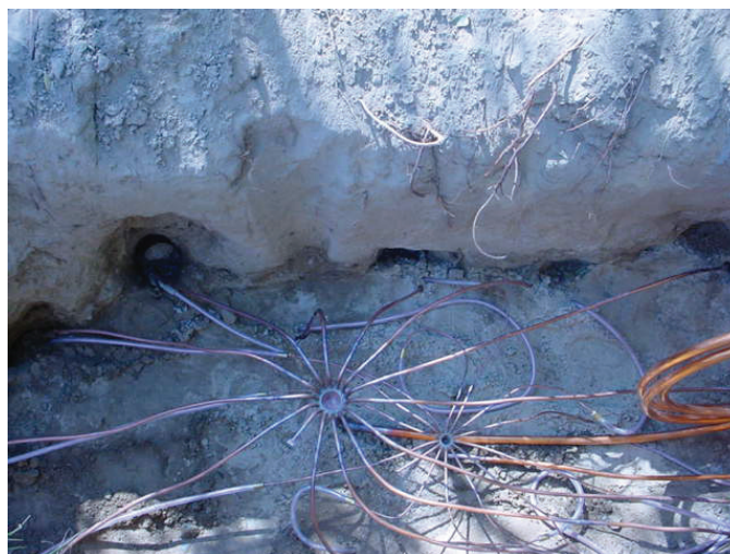
Figure 44.47 Diagonal earth-loop supply (liquid) and return (vapor) manifolds in a pit. Courtesy Earthlinked Technologies, Inc.
