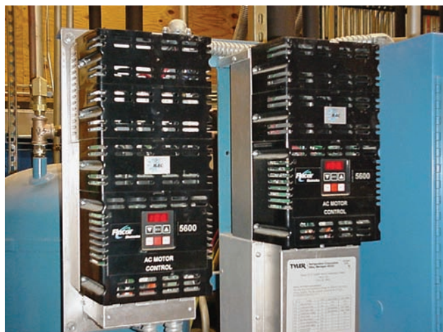
Figure 26.22 Inverters or variable-speed drives that change the alternating current's frequency, thus changing the satellite compressor's speed and capacity for better load matching.
