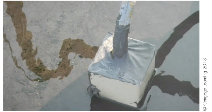
Figure 50.28 Pitch pockets are used when piping or conduits must penetrate the roof. Photo by Eugene Silberstein
