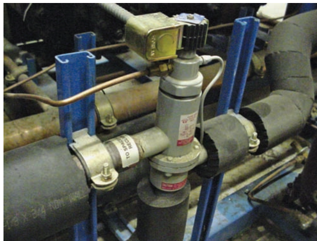
Figure 26.7 A heat reclaim valve shown mounted securely to handle any expansion and contraction forces.
