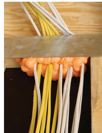
Figure 36.36(B) Insulating foam sealant sealing air leaks where electrical wiring penetrates through walls. Courtesy U.S. Department of Energy
