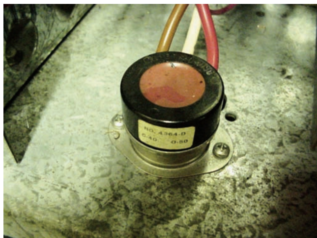
Figure 25.14(B) A thermal disk-type fan speed control. Courtesy Ferris State University. Photo by John Tomczyk
