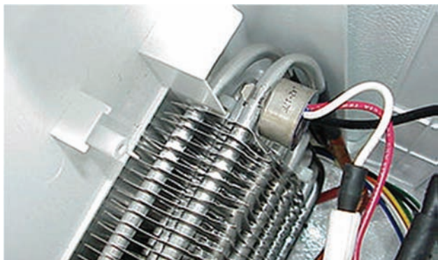
Figure 45.102 Defrost termination thermostat.
