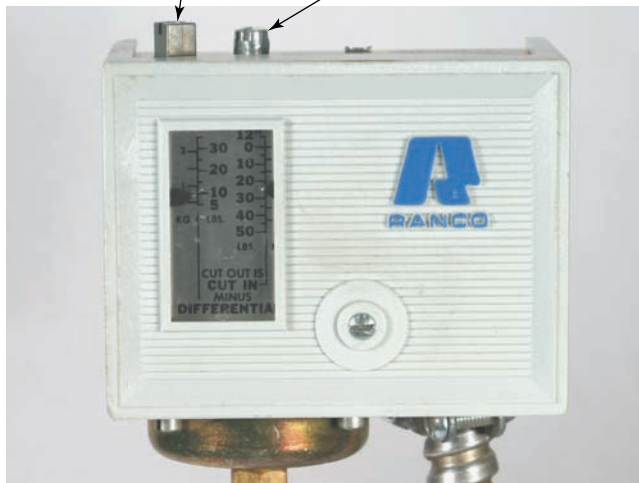
Figure 14.51 The low-pressure control. Photo by Bill Johnson
