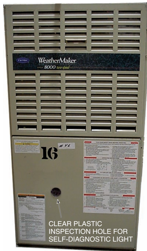
Figure 31.113 A furnace with a clear plastic inspection hole on the front panel for observing the self-diagnostic flashing light.
