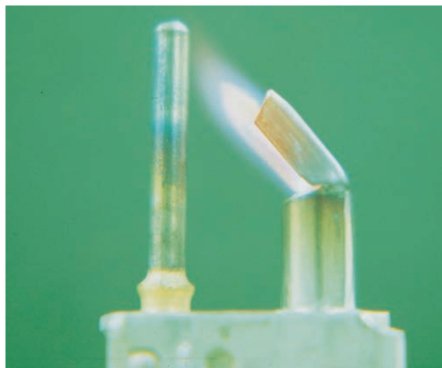
Figure 13.23 This thermocouple senses whether the gas furnace pilot light is on. Photo by Bill Johnson
