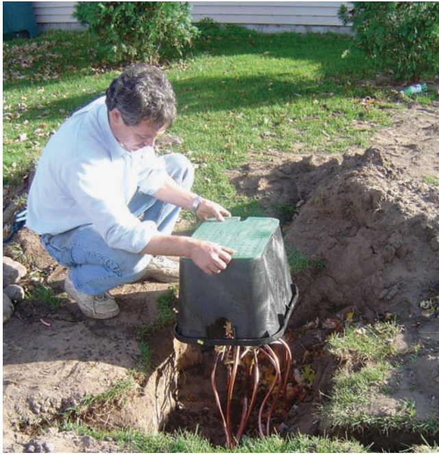
Figure 44.36 (Continued) (D) A header box being positioned over a copper header. Courtesy CoEnergies LLC, Traverse City, Michigan
