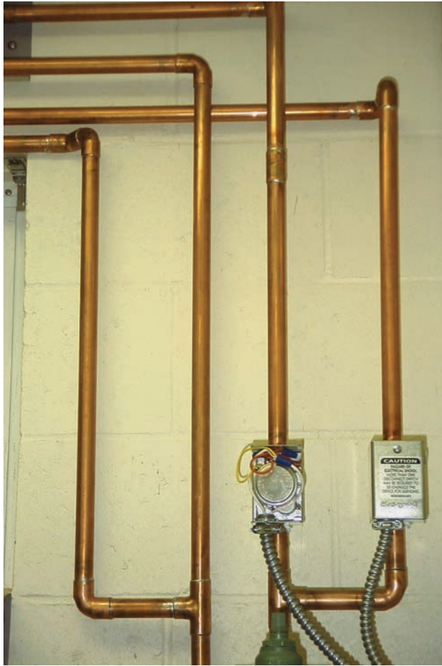
Figure 33.43 Gear motor zone valves on a multiple-zone loop. Photo by Eugene Silberstein
