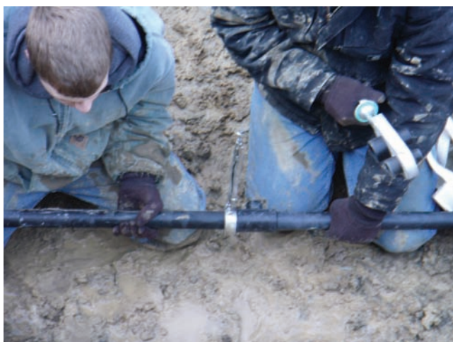
Figure 44.12(J) The plastic pipe and coupling tee being held together until they have cooled, in order to properly complete the heat fusion process. Courtesy Patrick Pung, Ferris State University HVACR Graduate
