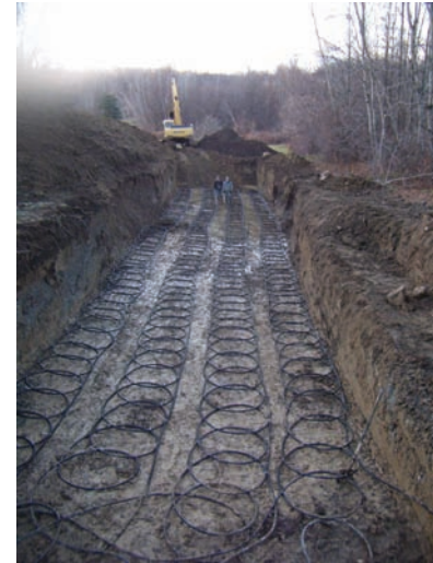
Figure 44.12(F) Freshly excavated trench showing four slinky ground loops with a large backhoe in the background. Courtesy Patrick Pung, Ferris State University HVACR Graduate
