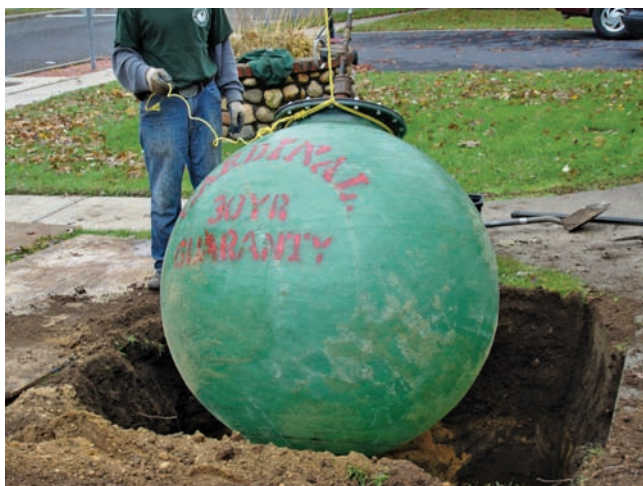
Figure 32.7 An underground fiberglass oil storage tank. Courtesy Oilheat Associates, Inc. Photo by John Levey
