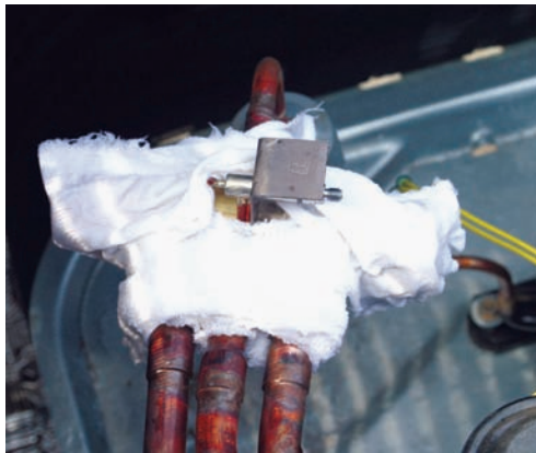
Figure 43.12 This valve body has a wet rag wrapped around it and water is dripped on the rag to keep the valve body cool. Photo by Bill Johnson
