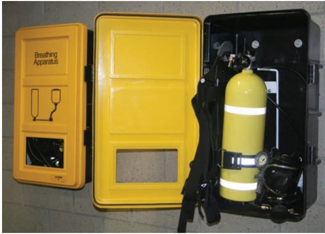
Figure 49.31 This breathing apparatus is mounted where a technician can easily reach it and put it on in case of a refrigerant leak alarm. Courtesy Ferris State University. Photo by John Tomczyk
