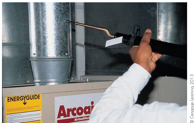
Figure 32.101 Making a smoke test. Photo by Bill Johnson
