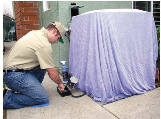
Figure 8.7 A service technician has covered the condensing unit with a sheet to serve as a barrier against any outside air movement before using an electronic leak detector. Never use a plastic cover because some plastics will set off certain electronic leak detectors and give a false reading. Courtesy Refrigeration Technologies, Anaheim, CA
