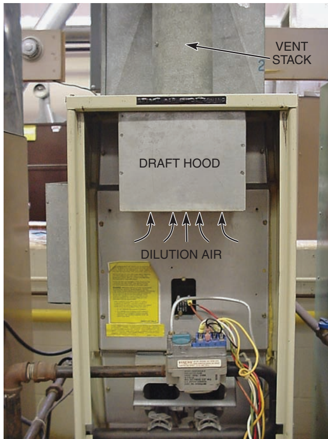
Figure 39.58(A) Dilution air is excess air after combustion and usually enters at the end of the heat exchanger. It is brought in by the draft hood of the furnace. Courtesy Ferris State University. Photo by John Tomczyk
