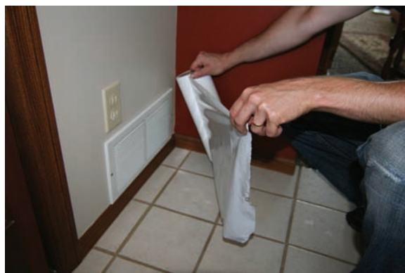
Figure 39.48(B) Tape off all return registers with a duct sealing material such as Duct Mast or a high-quality painter’s masking tape and masking paper. Courtesy Ferris State University. Photo by John Tomczyk
