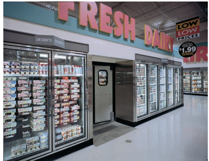
Figure 26.41 A display case with a walk-in cooler as its back wall. The display case can be supplied from inside the cooler. Courtesy Hill Phoenix
