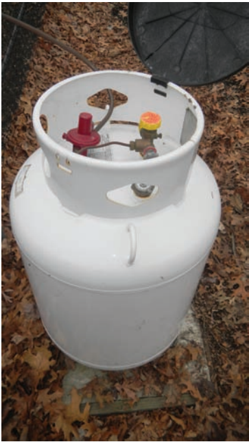
Figure 14.63 The gas pressure regulator on a bottled-gas system. This regulator is on the tank. Photo by Eugene Silberstein
