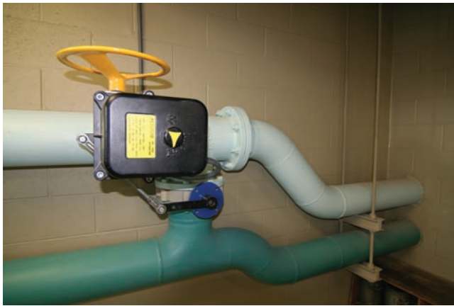
Figure 48.40 (A) A mixing valve application. (B) A direct digital controlled (DDC) butterfly valve bypass. The valve will bypass some of the warm water coming from the water-cooled condenser's outlet and mix it with cooling tower outlet water.
