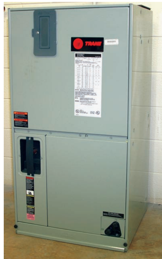
Figure 43.30 An air-to-air heat pump indoor unit. It is an electric furnace containing a heat pump coil. Notice that the air flows through the heat pump coil and then through the heating elements. Photo by Bill Johnson
