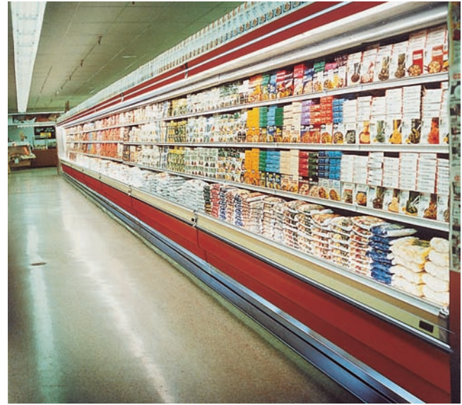
Figure 26.2 Open display cases maintain even, low-temperature refrigeration because cold air can be controlled. It falls naturally. Air patterns are formed to create air curtains for shelves that are up high. These air curtains must not be disturbed by the air-conditioning system's air discharge. All open cases have explicit directions as to how to load them, with load lines conspicuously marked.
