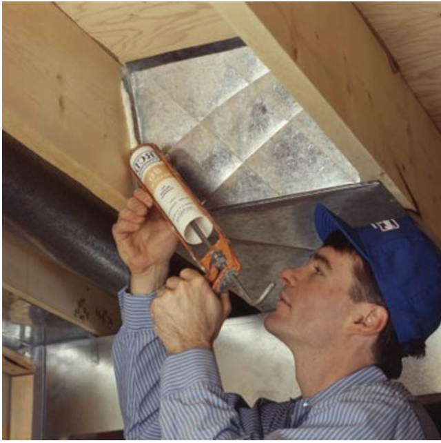
Figure 39.46(B) Seal all return-air cavities. Courtesy The Energy Conservatory
