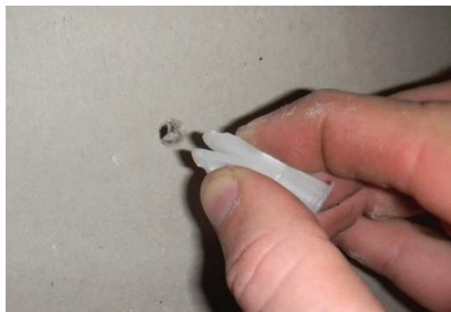
Figure 6.23 The folded plastic toggle inserted into the hole in the gypsum board. Photo by Eugene Silberstein
