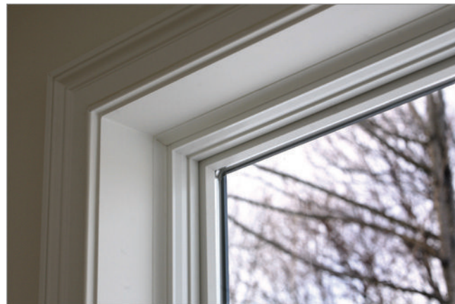
Figure 39.31(B) Gasket material between the window frame and the glass of a double-pane window. Thermal bridging can be lessened by installing a gasket material made of a poor thermal conductive material between the window frame and the glass. The gasket material is often referred to as a thermal break. Courtesy Fluke Corporation
