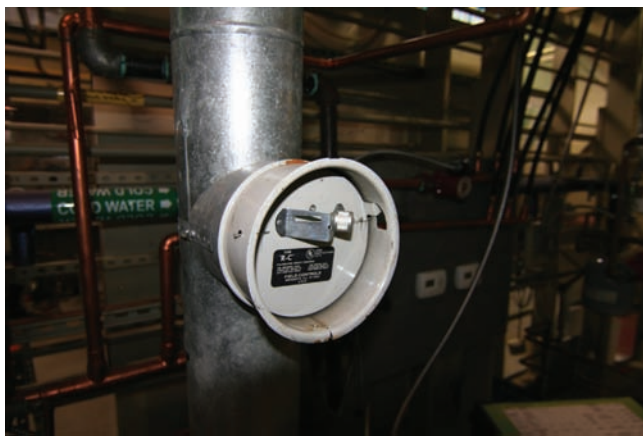
Figure 39.63 Barometric dampers are used to maintain constant over-the-fire drafts regardless of chimney or vent system draft conditions. Courtesy Ferris State University. Photo by John Tomczyk
