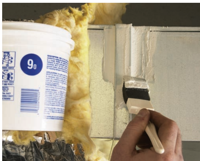
Figure 38.2 Technician applying mastic to a joint between two duct sections.
