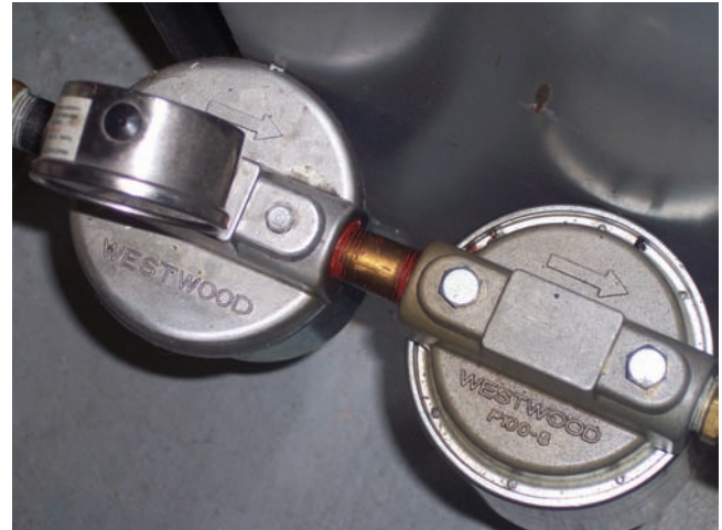
Figure 32.23 Make certain that the arrows on oil filters point in the direction of oil flow. Courtesy Oilheat Associates, Inc. Photo by John Levey
