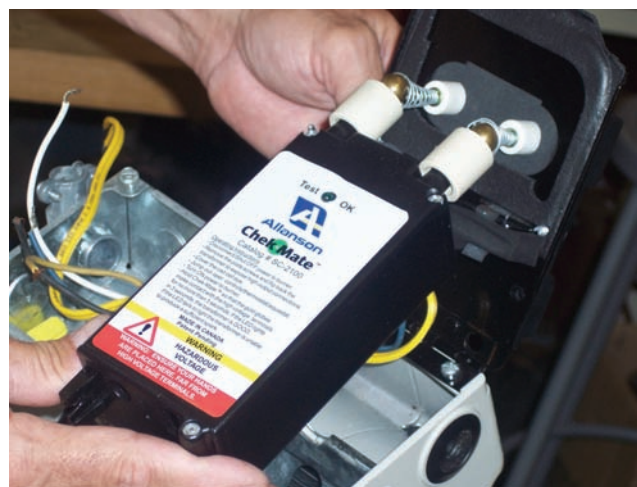
Figure 32.67 A solid-state igniter tester. Courtesy Oilheat Associates, Inc. Photo by John Levey
