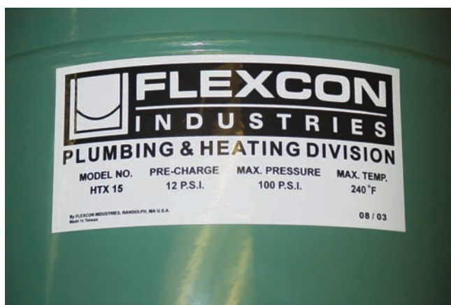
Figure 33.16 Expansion tank data tag. Photo by Eugene Silberstein
