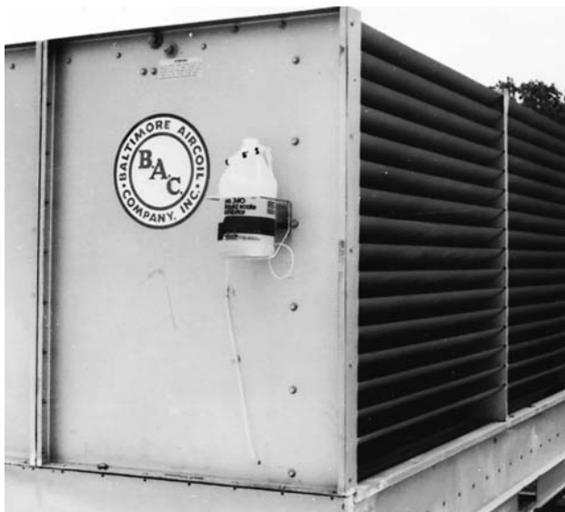
Figure 22.5 A method of adding water treatment to a cooling tower. Treatment is being metered at a rate that will last about a month so the operator will not have to be in the tower constantly. The tower water bleeds continuously to the drain to avoid an overconcentration of minerals in the water. Courtesy Calgon Corporation
