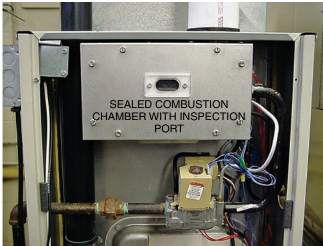
Figure 31.69 A sealed combustion chamber on a high-efficiency furnace. Courtesy Ferris State University. Photo by John Tomczyk
