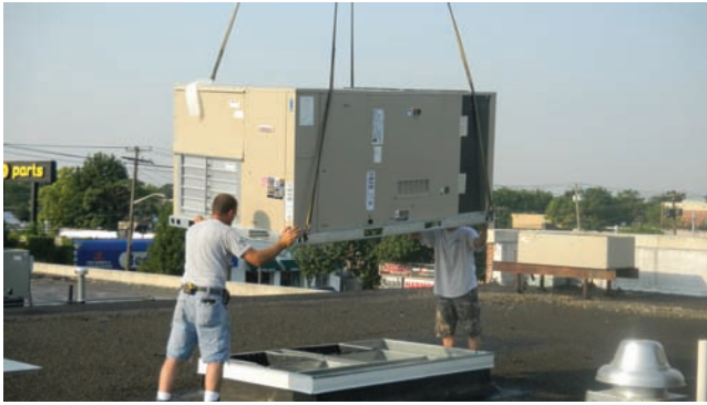
Figure 50.14 Two installation crew members guiding the unit into place. Photo by Eugene Silberstein
