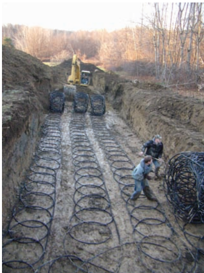
Figure 44.12(E) Technicians rolling out the last of four slinky ground loops. Courtesy Patrick Pung, Ferris State University HVACR Graduate
