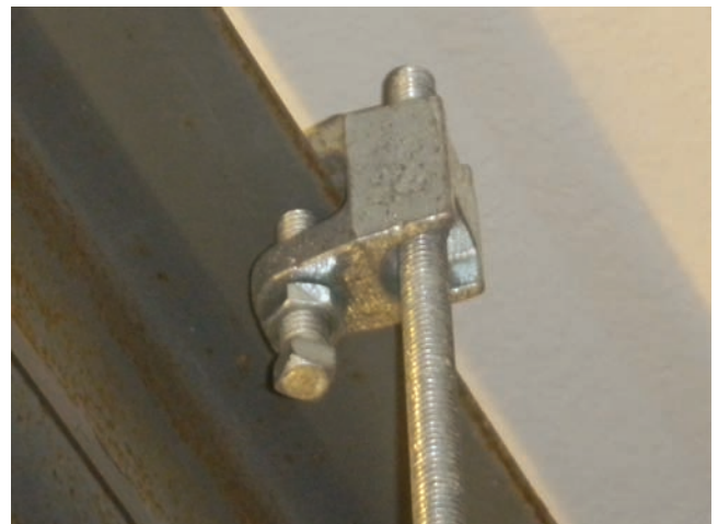
Figure 6.29 Beam clamp used to secure threaded rod. Photo by Eugene Silberstein
